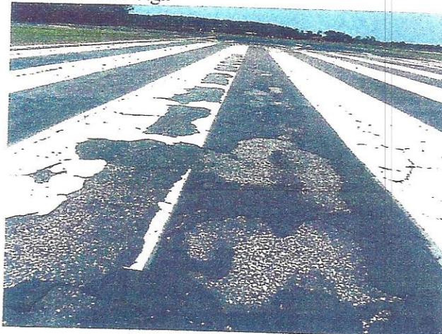
Pavement Breaking up
